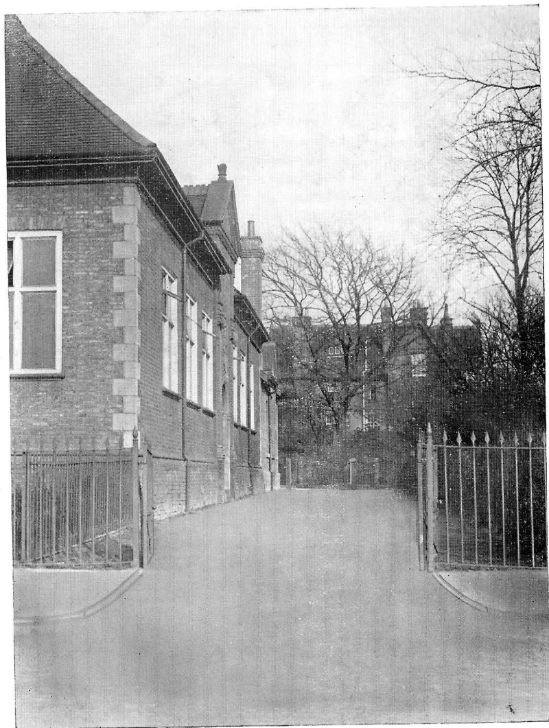
PART OF THE SCHOOL BUILDINGS
